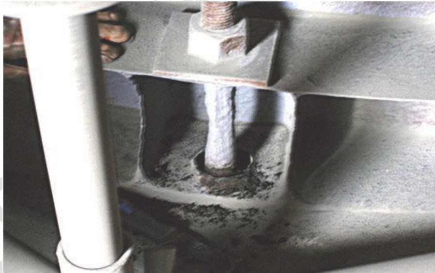
Figure B.18 - Corroded Anchor Bolting
