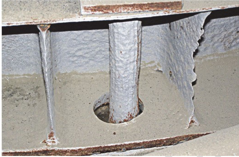
Figure B.17 - Corroded Anchor Bolting
